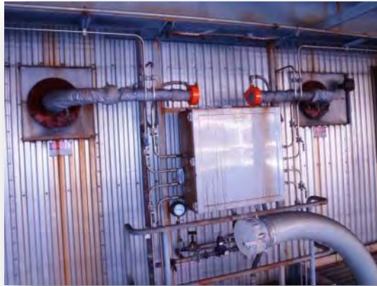
Sonic horns installed on SCR at Big Bend
